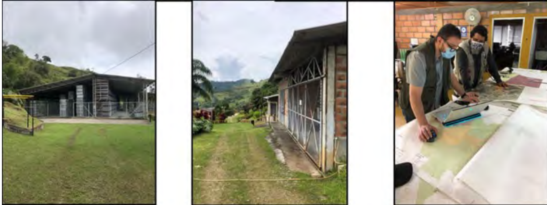
Figure 5.3. Drill core storage and core shed (left); workshop and supplies storage (central); detail of geology office (right) (Source: Mauricio Castañeda, QP, 2021)
